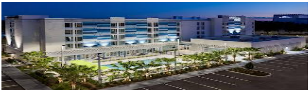
View of rear of Hotel
