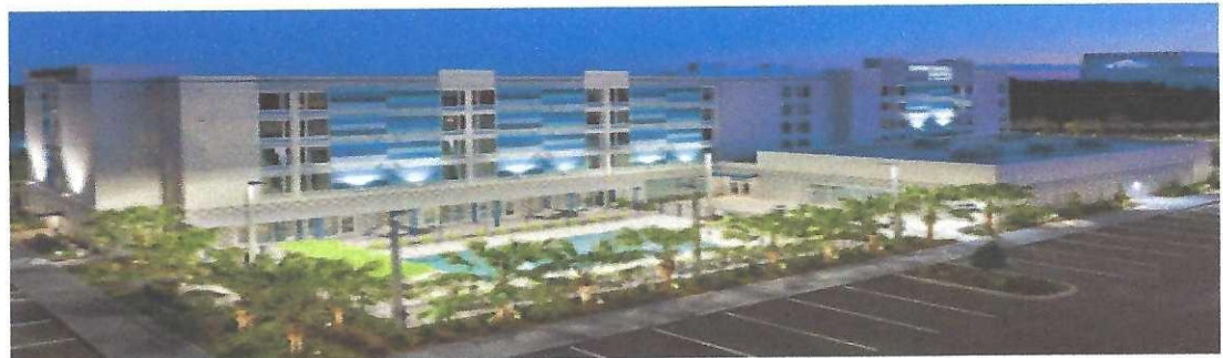
View of rear of Hotel
