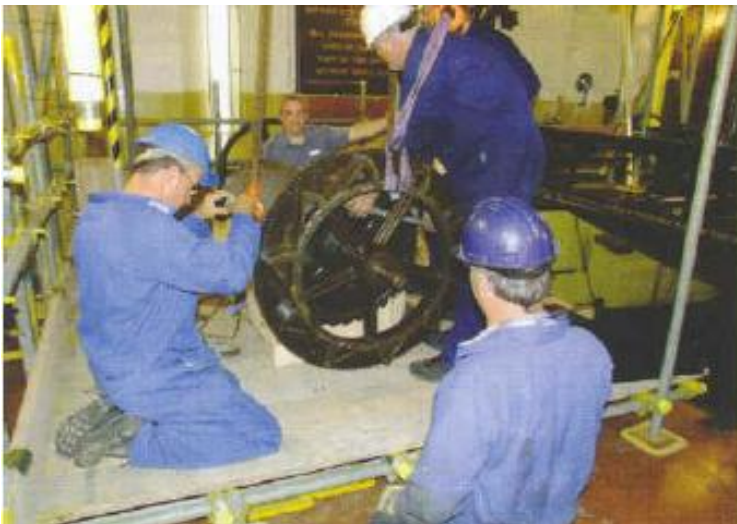
9. Safely in the cradle, the great wheel is removed from the barrel.
