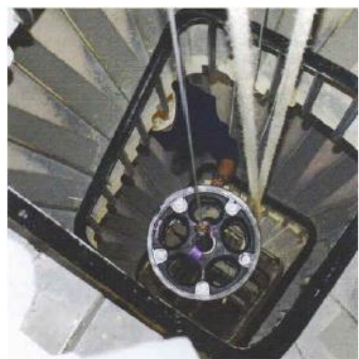
10. Strike barrel being lowered down the stair well.
