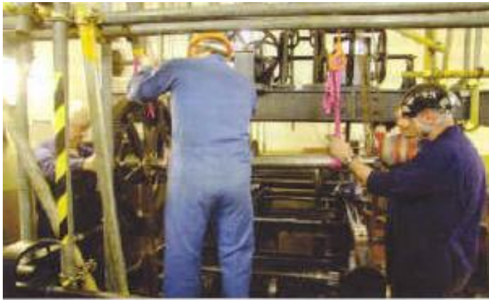
19. Strike great wheel and arbor being installed.
