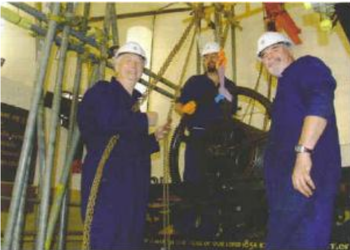
7. The Palace team lifting out the hour strike barrel
