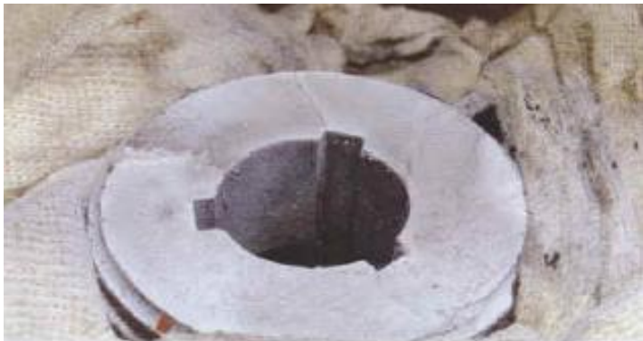
15. Cracks in going great wheel hub.
