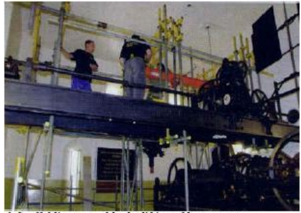
6. Scaffolding to enable the lifting of heavy parts
