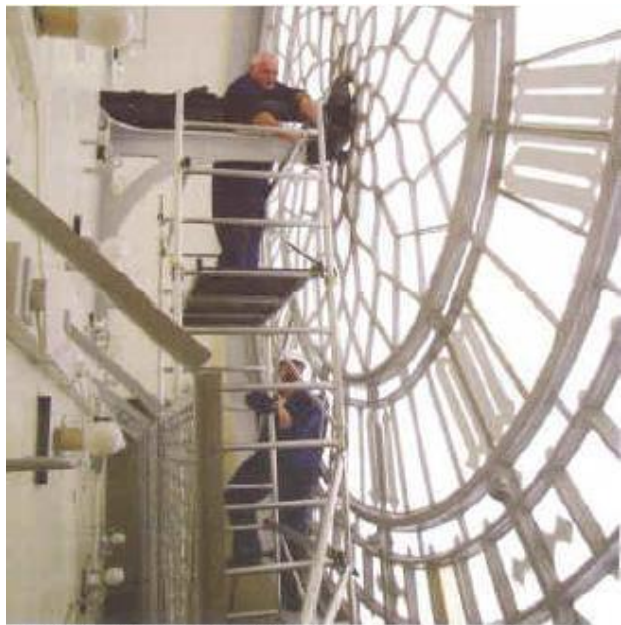
12. Scaffold to reach the 12 feet to the motion works.
