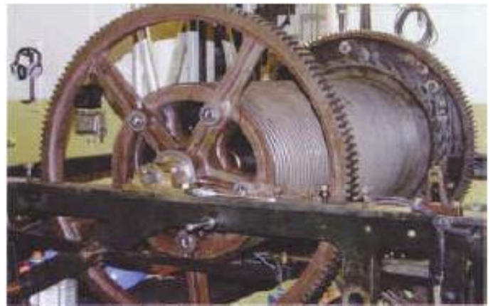
20. Strike wheel and barrel together and installed.
