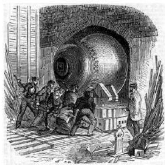
Big Ben bell on cradle being put into tower base
