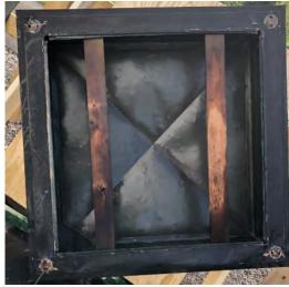
The top and bottom is copper which was badly bent and rotted and will be replaced with hand crafted copper top and bottom.
