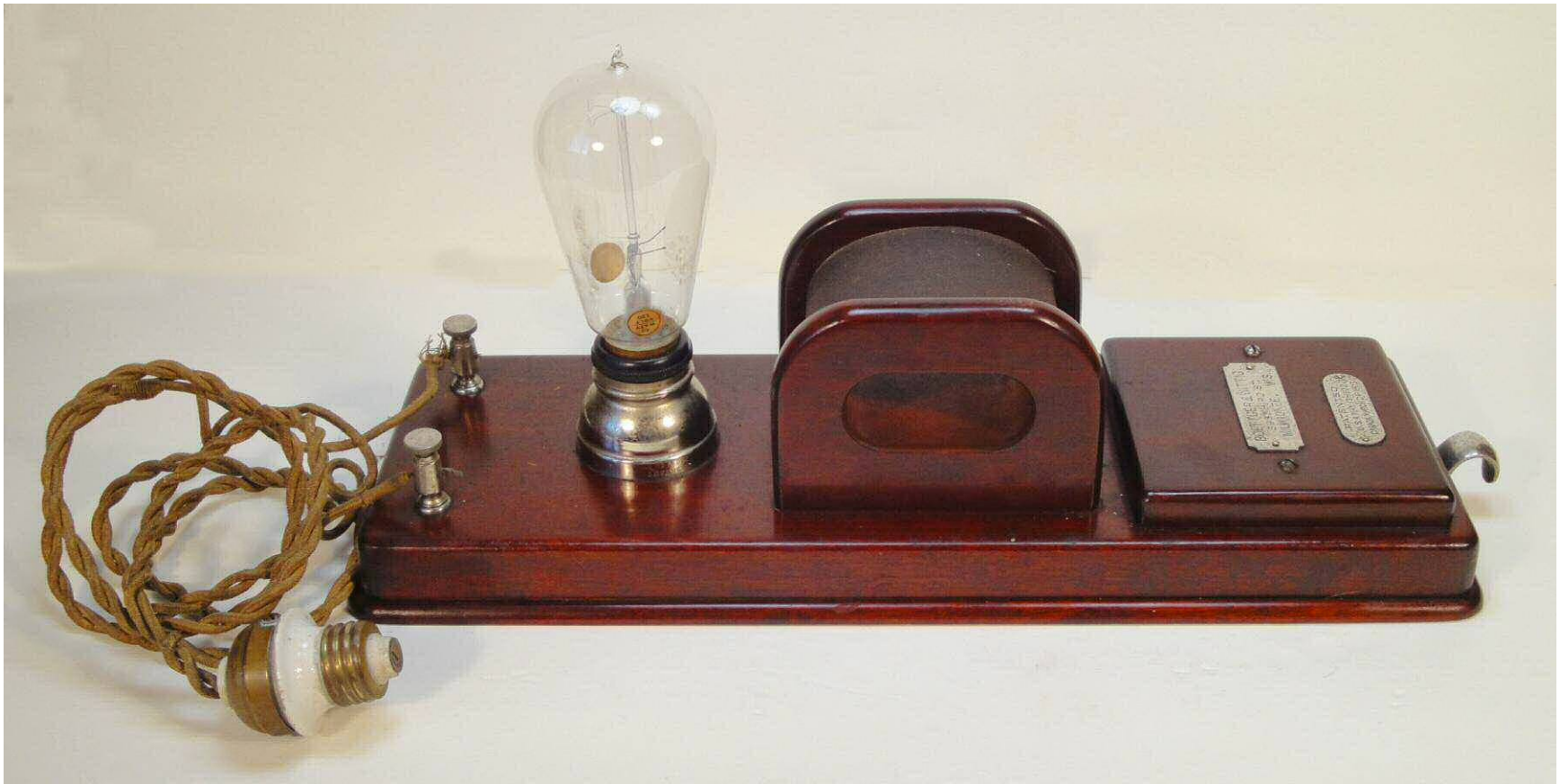
Boettger & Wittig Watch and Tool Demagnetizer made for both Direct and Alternating Current Systems.
