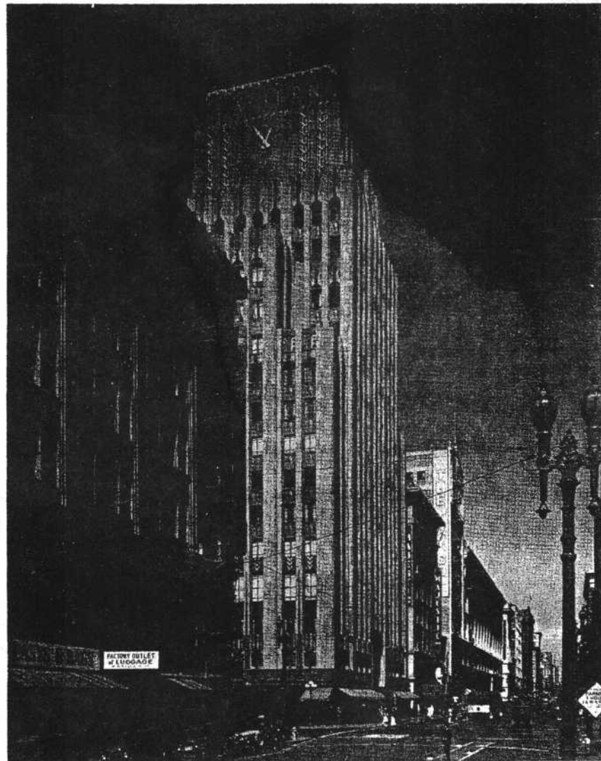
EASTERN-COLUMBIA BUILDING, Los Angeles, Cal. An ADFR (Automatic Double Frequency Resetting) Telechron Clock System is installed, consisting of four 15½ foot Neon illuminated tower clocks, twelve other specially designed clocks located throughout the interior of the structure and central control equipment. Installed September, 1930.
