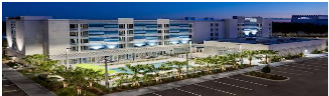
View of rear of Hotel
